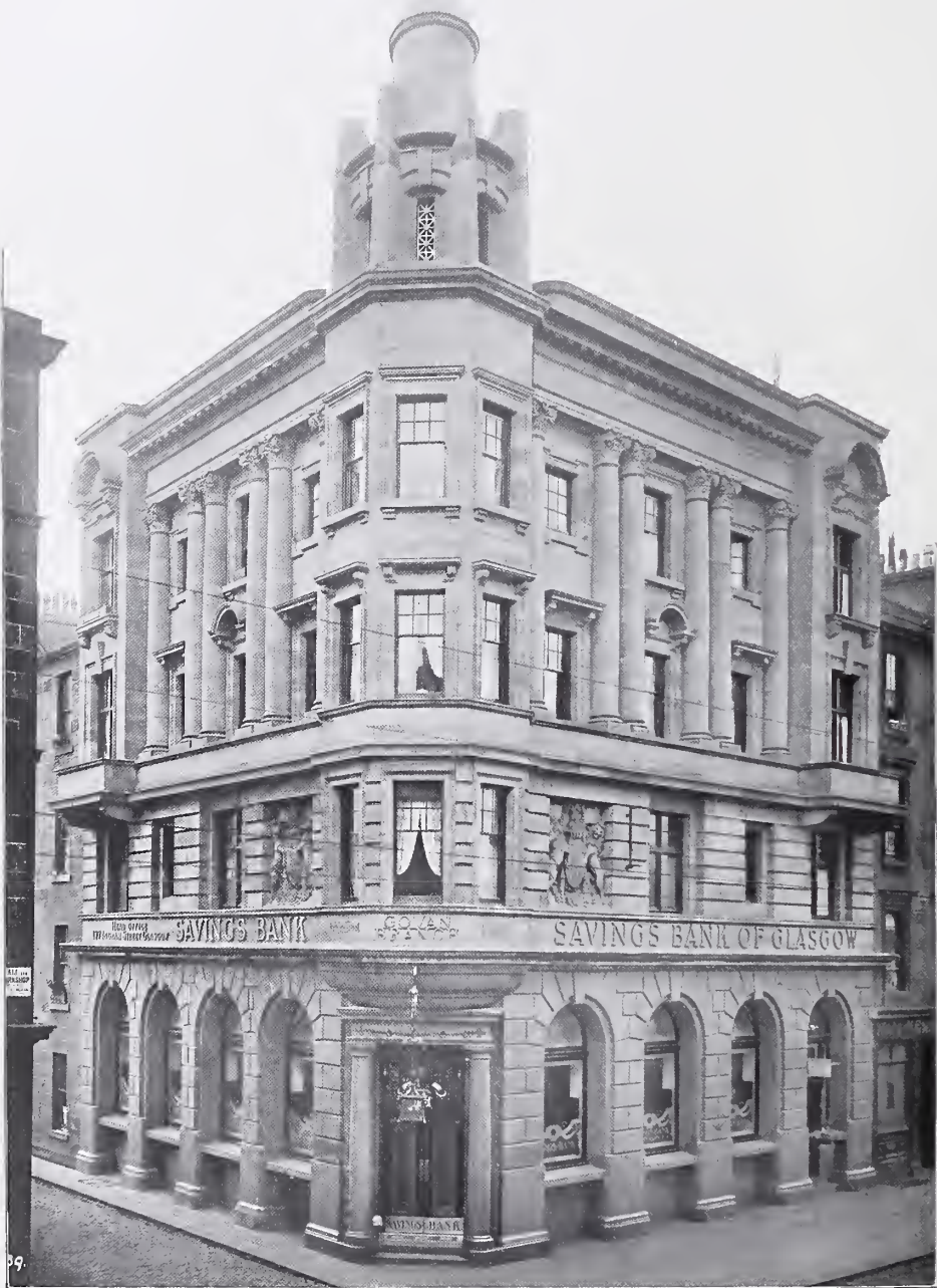
791. Savings Bank of Glasgow, Govan Branch, ERIC A. SUTHERLAND, Architect. Mason: G. Barlas and Co., 13 Ruthven Street, Hillhead, Glasgow. Joinery: John Cochrane, 58-70 Dobbies Loan, Glasgow. Marble: Galbraith and Winton, 185 St. Vincent Street, Glasgow. Heating: Cameron and Co., Glasgow.
